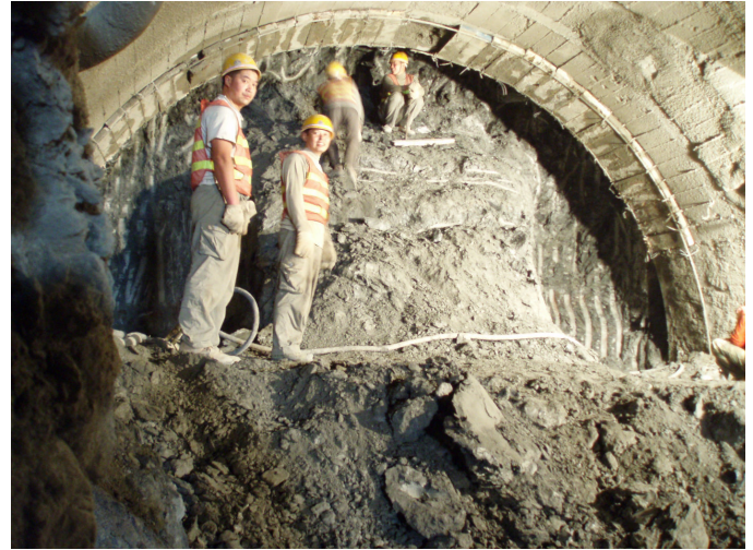
Figure 6. Construction of Ras R'Mel tunnel (Guiloux et al 2008).
