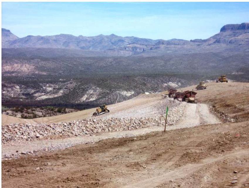
Photo 4: Installation of rock armor on 6 Dam
