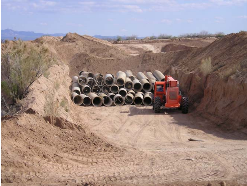
Photo 3: Transite pipe disposal in asbestos landfill
